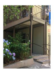
The major entrance to the 600 building complex between 600A and 600B appears to be inaccessible to anyone with a mobility problem, due to the steps that approach the elevator. Without directional signs, you have no clue that if you wind around behind the structure you can get to the elevator and save many steps if you need to go upstairs in 600A or 600B.
